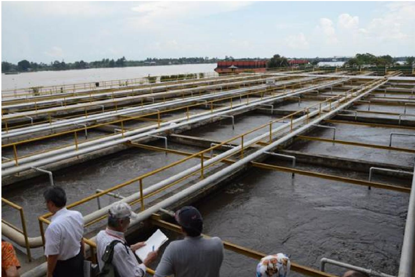
WWTP in PT.ABP
